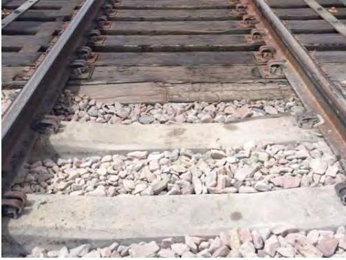
Fig. 7. Crib ties (top); concrete bridges (bottom).
